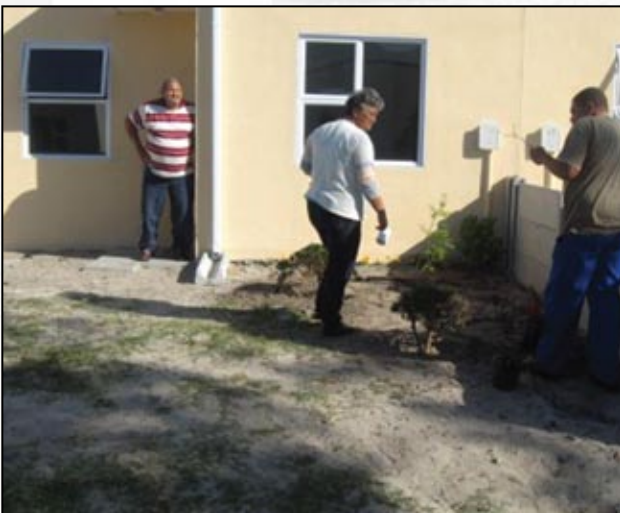
Light Steel Weight Building Technology in progress
