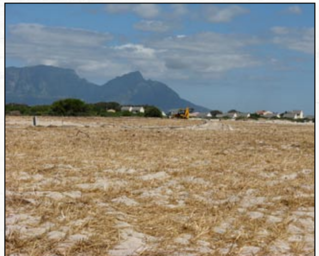
Land being cleared for future development, Morgan Village III
