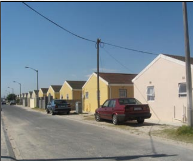
Housing complete in Luyoloville
