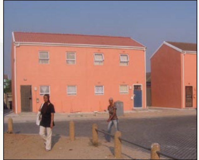
Eastridge Rectification Programme Completion
