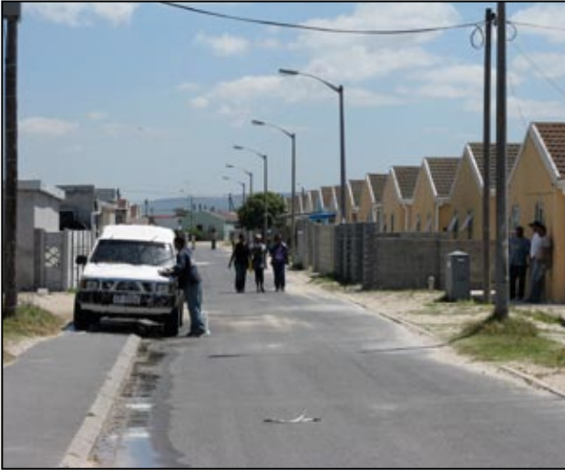
The Woodbridge development after the completion of the rectification process.
