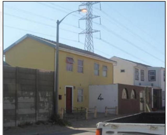
Housing complete in Pylon
